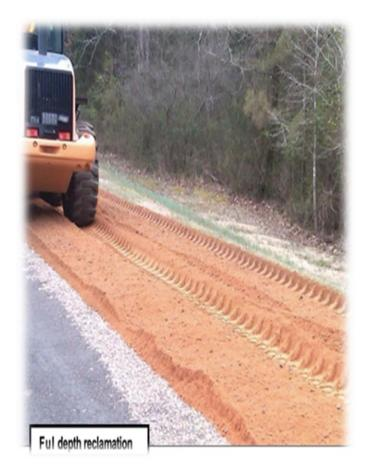
Full-depth reclamation uses the materials from the deteriorated asphalt pavement, and, with the addition of cement, creates a new stabilized base.
